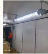
Installation Explosion Proof Air Conditioner & Explosion Proof Lighting
