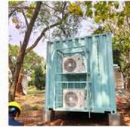
Installation Explosion Proof Air Conditioner & Explosion Proof Lighting
