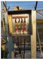
Installation Explosion Proof Junction Box Stainless Steel
