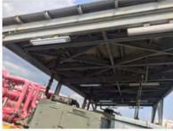
Installation Explosion Proof Lighting
