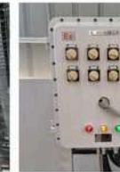
Installation Explosion Proof Junction Box Aluminium Alloy
